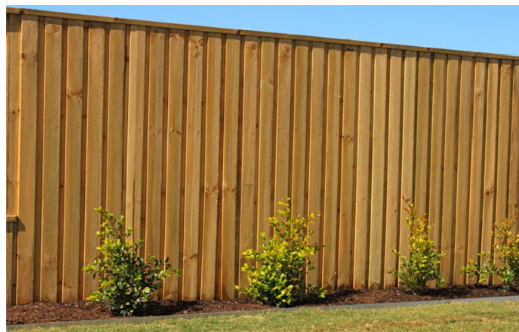
treated pine lap and cap fence: height 1.8 m
