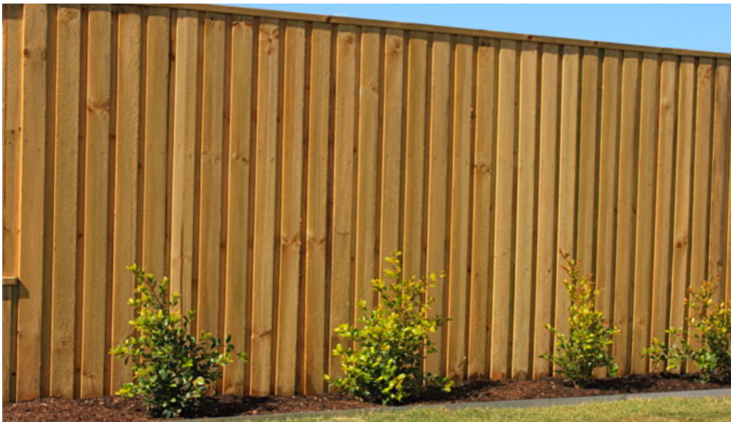
treated pine lap and cap fence : height 1.8 m
