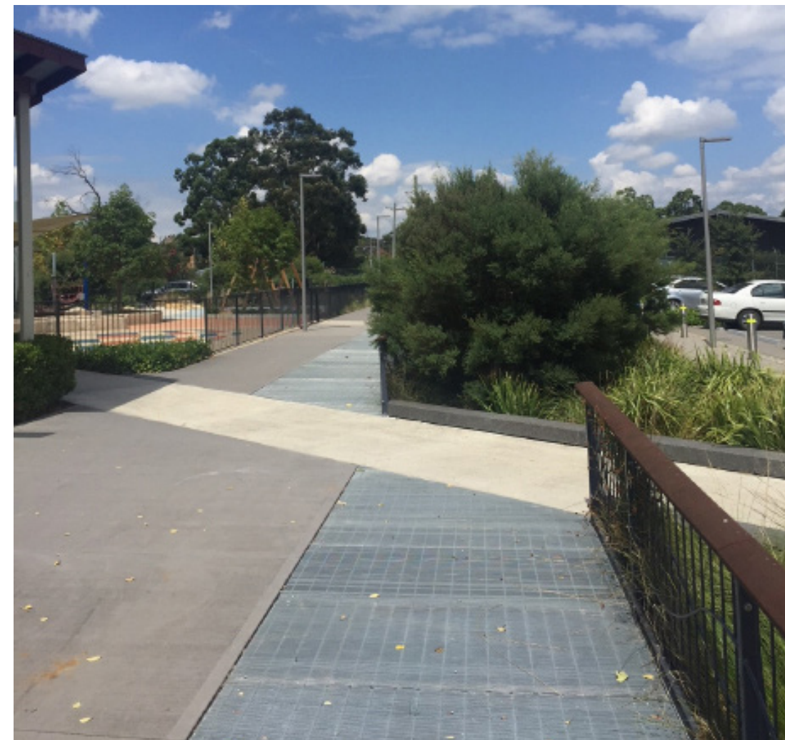
perforated FRC deck over Bio swale
